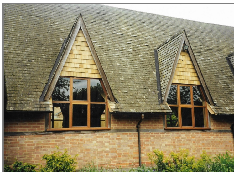
Hall windows before and after
