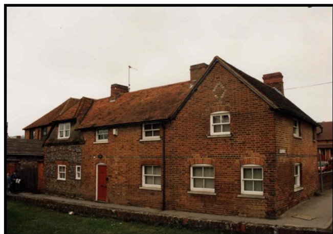
Old Gundy brew-house and buildings in Goring
