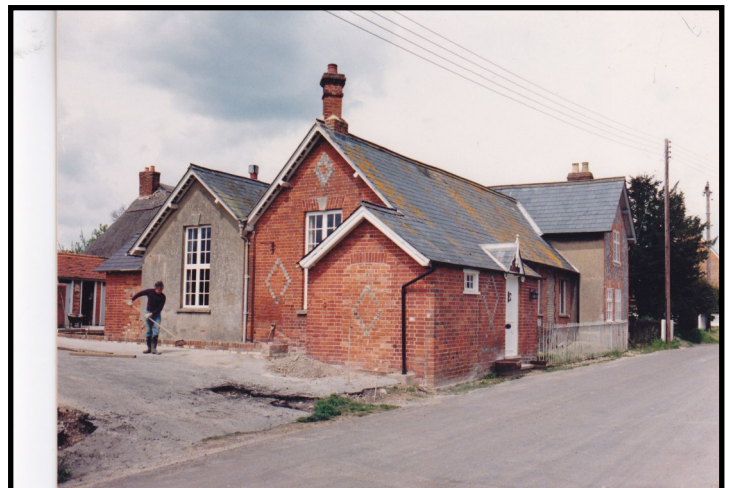
John Twine working on the Old School House
