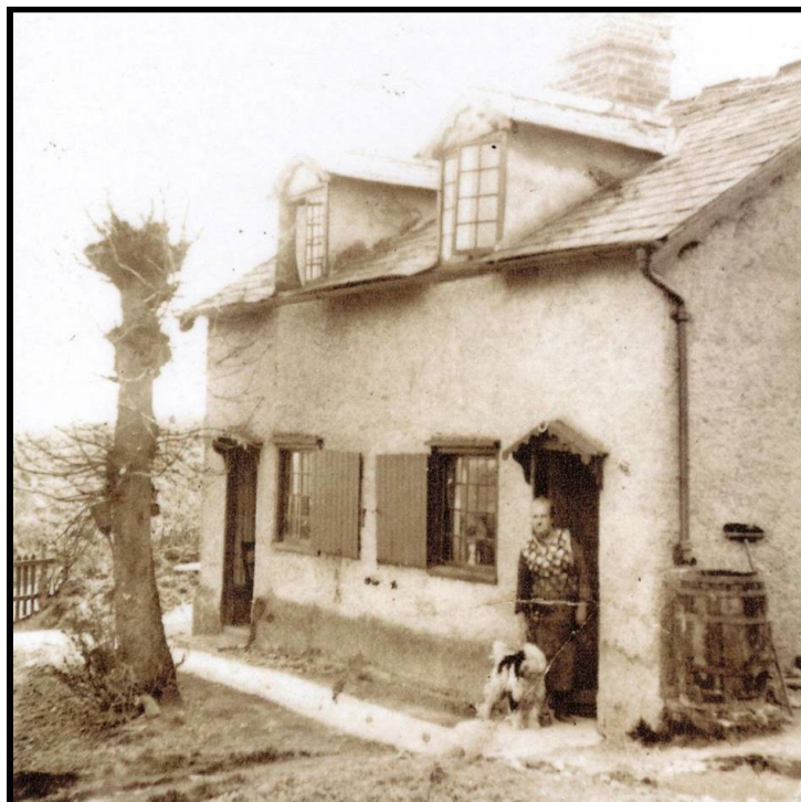
A photo of Chalk Hill Cottage, taken in the early 20th century.
